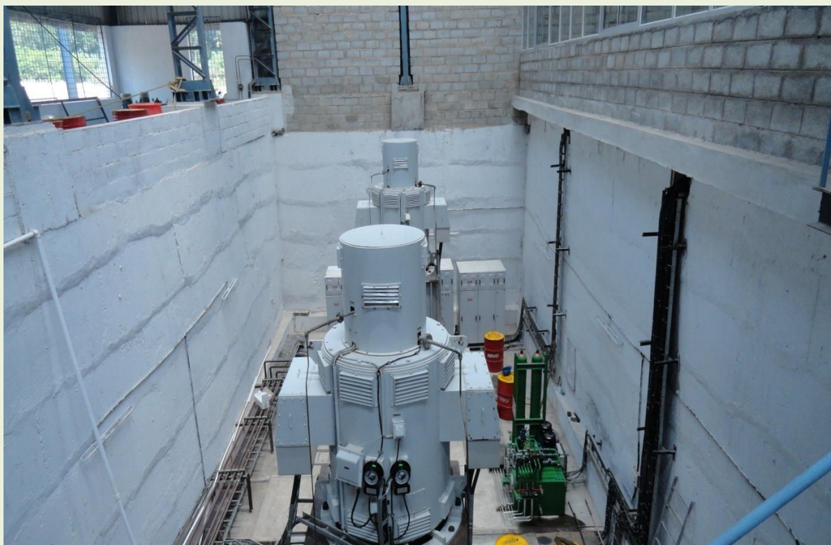
Kaplan Turbine Assembly
